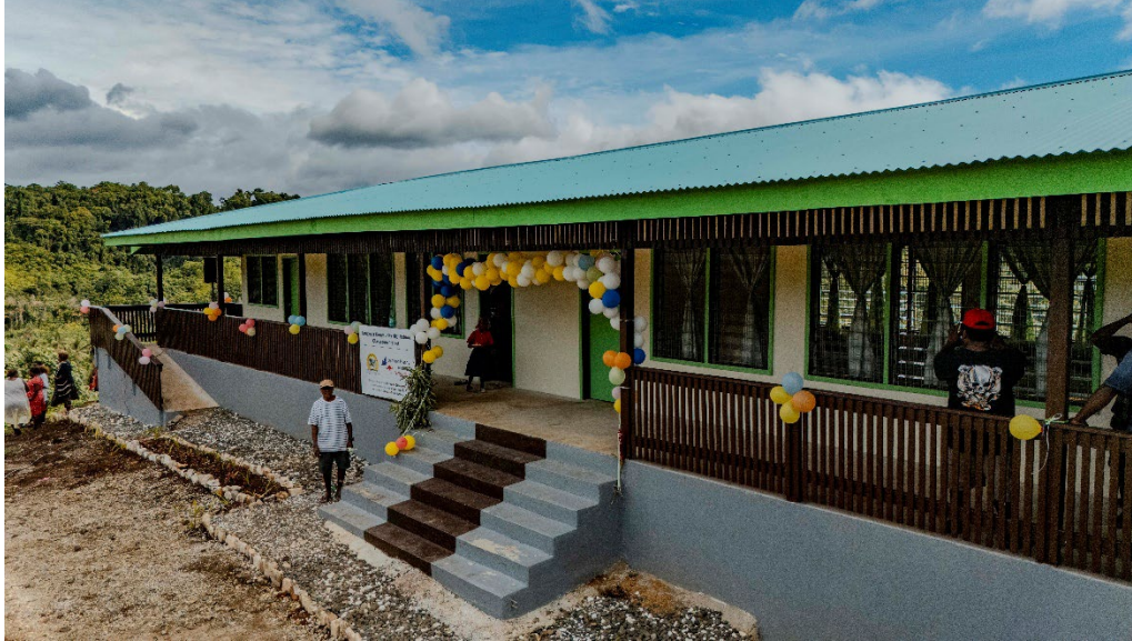
Caption: The new classroom building at Laugwata CHS contains three classroom and an office space.
